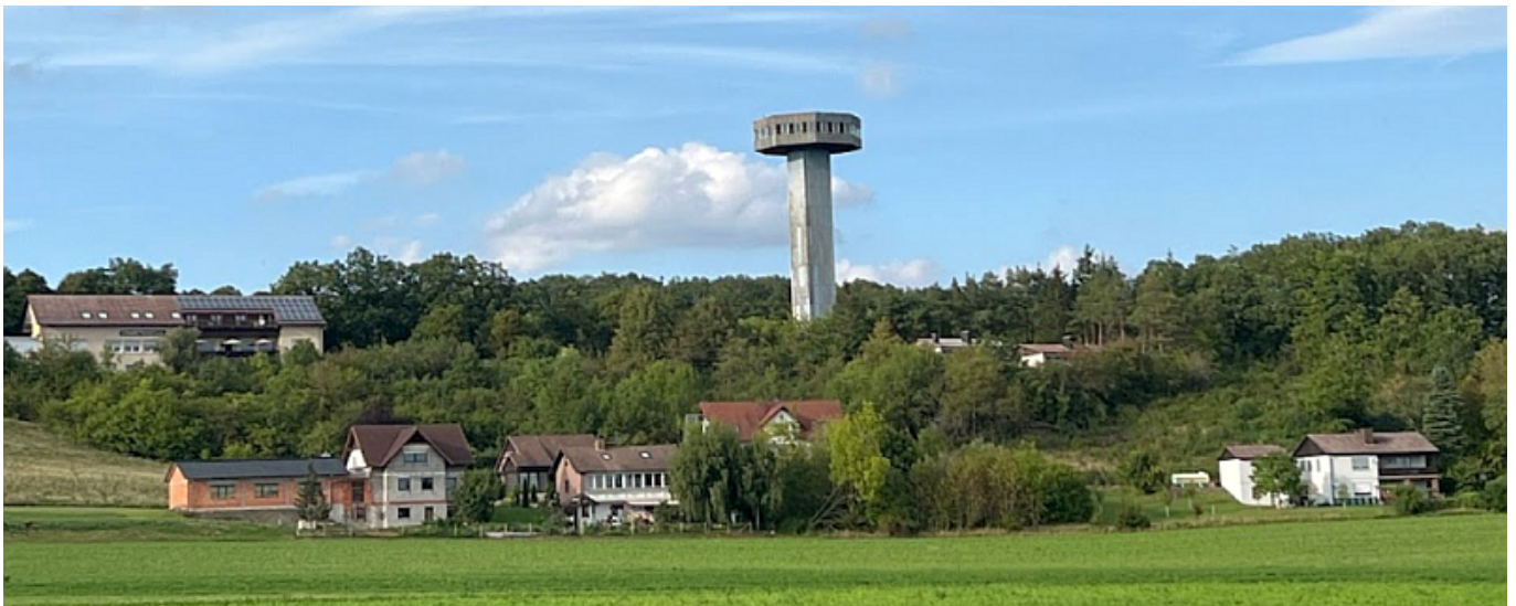
Bayernturm, the disused watchtower
